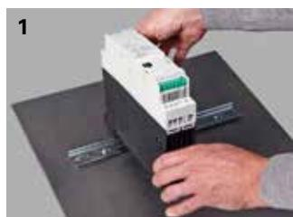
Snap the speed starter onto the top-hat rail.
